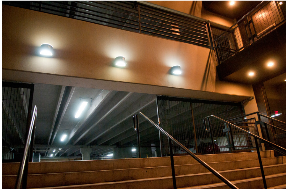
figure 2. Acropolis parking garage, downtown Albuquerque, NM
