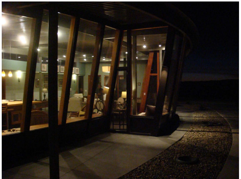
Exterior of the Wyatt residence.
