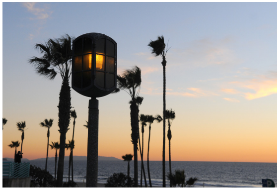
One of the many lantern fixtures along Manhattan Beach Boulevard retrofitted with Norbach LEDs.
